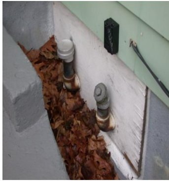
Vent pipes needs to be extended higher
