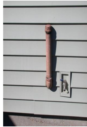
Vent pie is 6' higher than fill pipe but may be Restricted by siding
