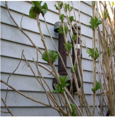
Vent pipes needs to be extended higher
