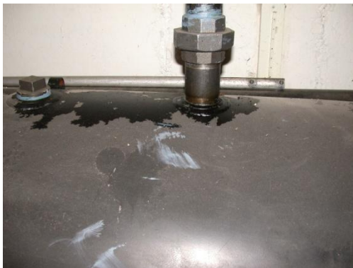
Both pictures above show leaking pipe threads
