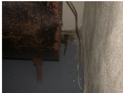
Abandon Tank in basement
