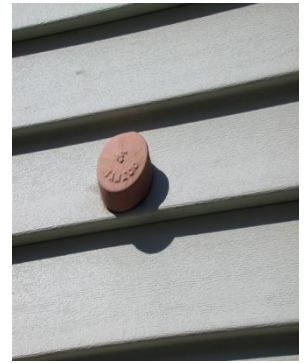
Vent pie is 6' higher than fill pipe but may be Restricted by siding
