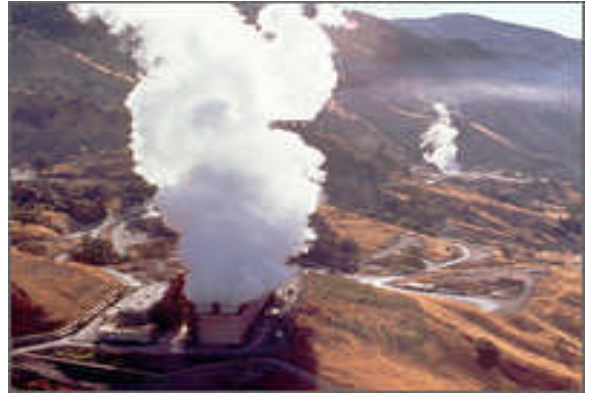
Several geothermal power plants at The Geysers.
